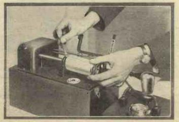
The sensitised paper is secured to the cylinder by means of a clip
