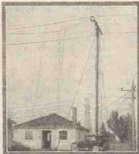
The transmitting hut and aerial of 2XAD, the Schenectady relay of the G.E.C., which transmits on 15, 22 and 26.8 metres
