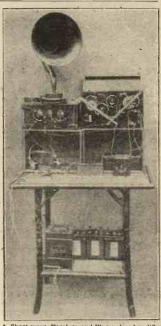
A Short-wave Receiver and Five-valve Amplifier made by Mr. H. G. Ede (Islington) from instructions in the "Work" Handbook "Wireless Telegraphy and Telephony."
