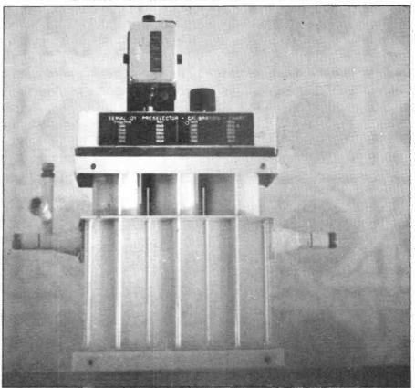
Tunable bandpass filter covering 1250-1350MHz (bandwidth 5 to 8MHz), obtained at a Leicester rally.
