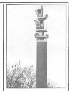
Height is important for VHF, UHF and microwave antennas — hence the tower!
