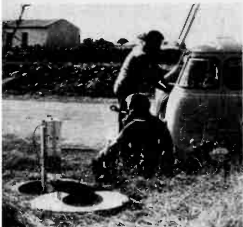
European engineers of the International Telephone and Telegraph Corporation install a buried transistor repeater for a carrier telephone system in Sardinia, using a new type of coaxial cable that is thinner than a pencil.
