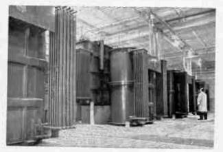
Fig. 2. Bank of high voltage transformers and rectifiers for supplying 120,000 volt DC power to transmitter. Photograph shows units undergoing test at G.E.'s high power radar laboratory, Syracuse.
