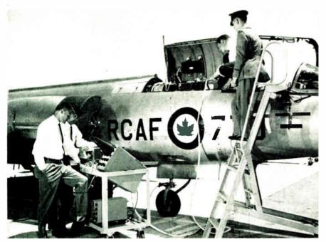
NEW PROOF OF LITTON'S CONTINUING CONTRIBUTIONS TO THE DEVELOPMENT OF INERTIAL NAVIGATION IS FURNISHED BY THE LN-3-2B AUTOMATIC NAVIGATOR THAT IS NOW BEING INSTALLED IN CANADA'S CF-104 FIGHTER.
