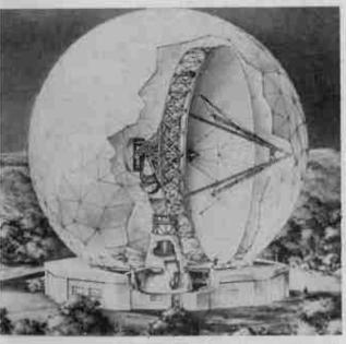
Artist's conception of USAF's Haystack Hill Radio Research Facility, Tyngsboro, Mass., slated to be the most powerful in the world through use of 100,000 watt plug in transmitters being built by Radiation at Stanford under \$1.6 million contracts.
