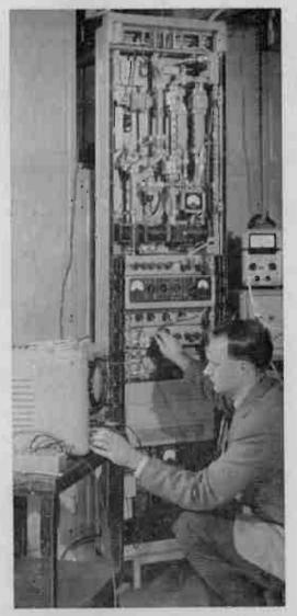
Engineer in General Electric Company Ltd. of England. Coventry, tests prototype super high frequency radio equipment of the type which will be supplied for a broadband radio link between Moncton, New Brunswick and Gore, Nova Scotia. This link will consist of two terminals and two repeater stations, and will form part of the Canadian east coast microwave network.
