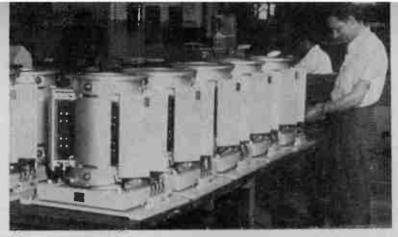
Over 3,000,000 digital bits will be stored on these computer memory drums avaiting installation at Ferranti-Packard Electric Ltd. The rotation of these drums may be phase locked to simulate one large drum, 10" diameter and 60" long.
