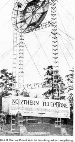
Collins Radio Company of Canada, Ltd. for Northern Telephone Company's Kenora-Red Lake system. Equipment includes Eimac Type 3K3000LQ klystrons, and Type 3X100A5 driver tubes... provides up to five toll quality voice channets.
