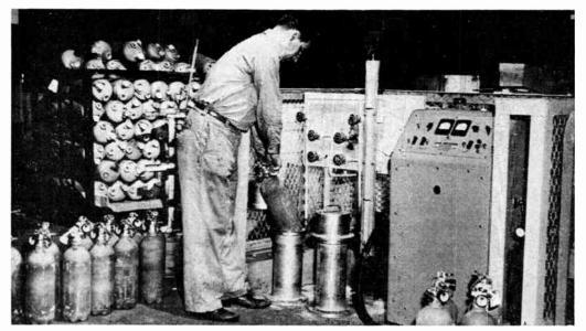
• Using Leak Detectors at Walter Kidde & Co. plant for leak-inspection of fire extinguisher cylinders,
