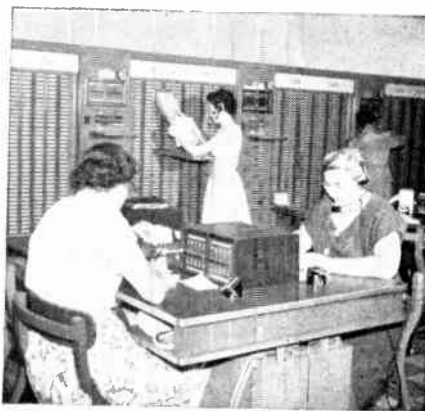
A new dial PBX system facilitates the handling of a greatly increased volume of calls. Shown here is part of the special customer contact service which required 24 positions of special answering equipment.
