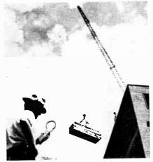
The Handie-Micro-Talkie transmitter may be used with any standard F.M. mobile set or base station operating on the same frequency. Subminiature dry battery power supply uses standard 30 and 1.5 volt cells, providing up to 30,000 ten second transmissions on a set of "B" batteries; up to 15,000 ten second transmissions on a set of "A" batteries. There is no stand-by current drain, power is consumed only while transmitting.
