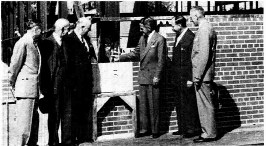
● Mr. W. H. McFadzean, Chairman of British Insulated Callender's Cables is shown tapping the corner stone in place, for the new buildings of the Phillips wire and cable company in Brockville. Mr. T. A. Lindsay, President of Phillips placed a cache of 11 modern cables in a crypt behind the stone, which were all suitably labelled for future generations to discover. Left to right: Mr. J. R. Phillips and Mr. A. Lauder, Vice-Presidents; Mr. H. F. Akehurst, Overseas Manager BICC; Mr. McFadzean, Mr. Lindsay, Mr. F. W. Barnhouse, General Sales Manager.
