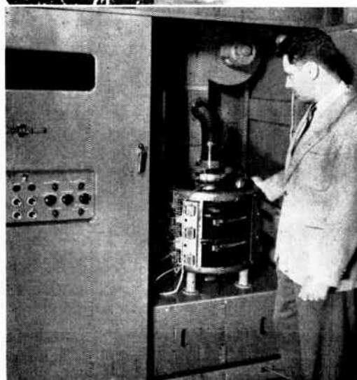
Collins two and ten kilowatt forward-scatter transmitters utilize Eimac amplifier klystrons, negative grid tubes and rectifiers.
