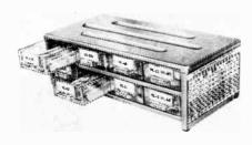
All piston capacitors in the PK85 are individually packaged, and housed by a rugged metal cabinet with a double row of compartment drawers.
