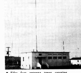
Fifty foot antenna tower carrying three special type antennas supplied by Rogers Majestic Electronics Limited.
