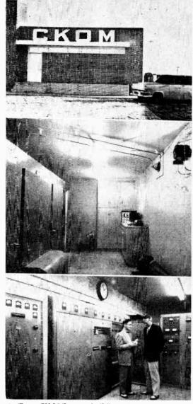
• Top: CKOM's new building. Center: Rear view of transmitter showing "deadback" construction. Bottom: Mr. Forst, and R. A. (Bob) Hosie right, examine the tube that delivers the stations 5000 watts.
