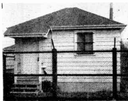
● The exterior of the receiving station at Point Grey, near Vancouver. This is a ship-to-shore receiving station.
