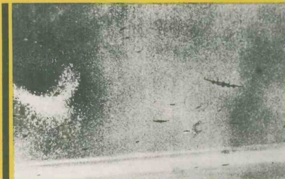
Strips of aluminum foil were dropped from aircraft to jam enemy radar. The strips were cut to a small size, but returned as much radar signal as an entire aircraft.
