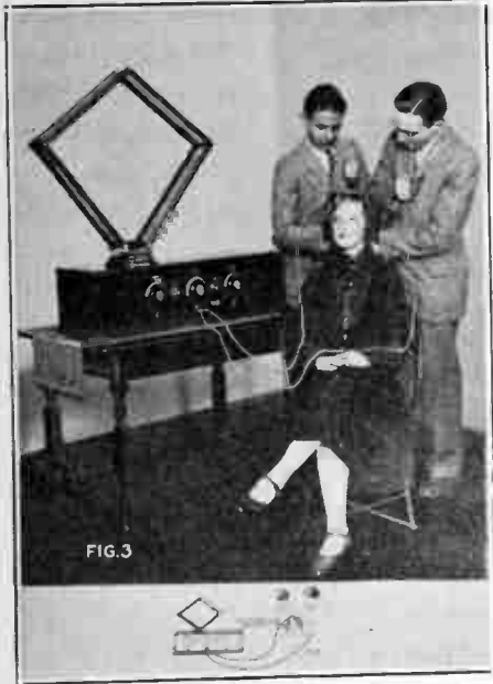
Fig. 3—When kid gloves become a radio head-set. In this experiment, the performers grasp the two bare wires coming from the radio set, while their gloved hands are held over the listener's ears. She will hear the sounds as well as with a regulation head-set. Fig. 3A shows how to make the connections.
