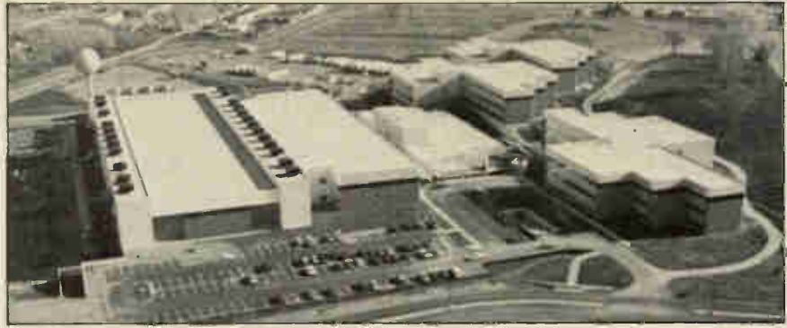
Seven-building $70 million data-processing complex recently opened by McDonnell Douglas. The 450 ft. long computer centre is at left.
