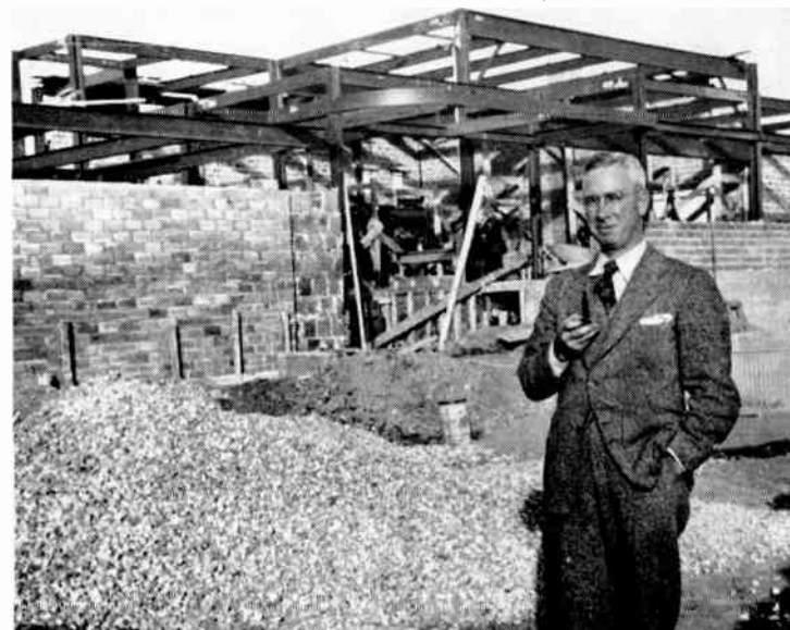
Chief Architect D. G. McKinstry photographed at CBX, Lacombe, Alberta, new CBC 50 Kw. transmitter building.
