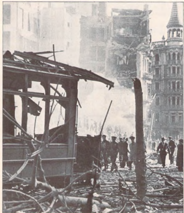
RAVAGES OF WAR: THIS SCENE OF RUIN IN BARCELONA WAS ECHOED ALL OVER SPAIN DURING THE BITTER 33-MONTH CIVIL WAR
