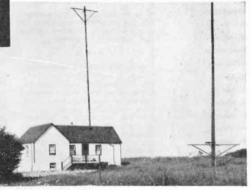
THE SEEDLING! CFRB's first transmitting station at Aurora. Ninety-eight feet high., wooden towers...
