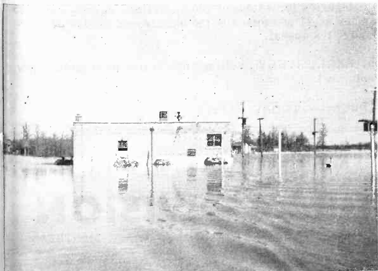
The CKRC transmitter at St. Vital which had to be abandoned.
