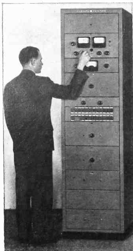
G.E. Cabinet Rack Type FA-8-A Showing Typical Audio Units Installed
