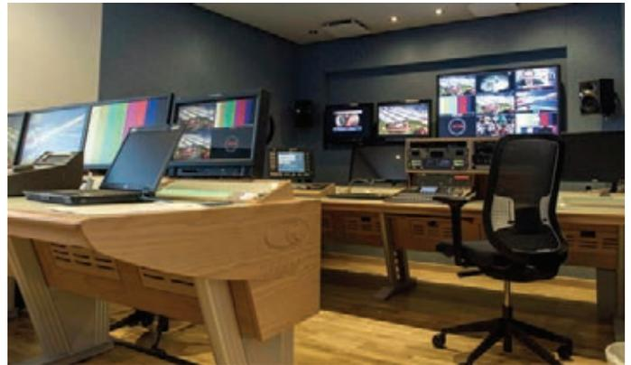
Input Media included Custom Consoles Module-R furniture as part of a major technical upgrade at its sports production studios in west London, with two V-shaped units providing eight operator positions at the front and nine and the rear.
