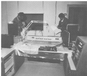
Jean-Claude Savoie and Rob Wreford wire the two-track production centre.
