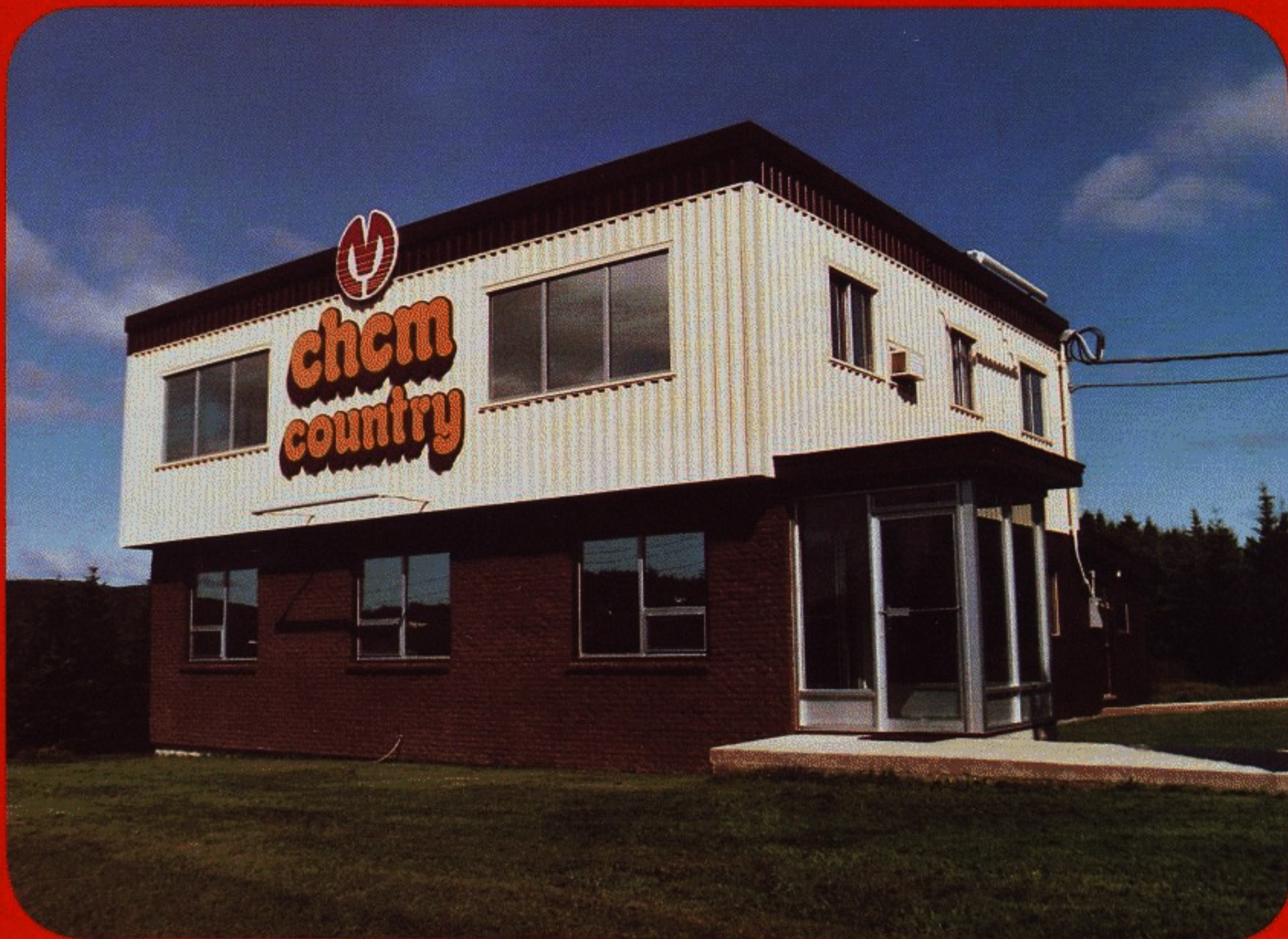
EXPANDED FACILITIES AT CHCM MARYSTOWN, NEWFOUNDLAND
