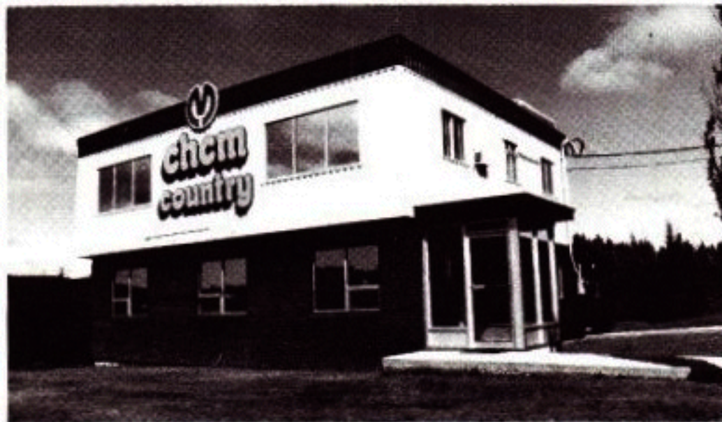
Exterior of expanded CHCM studio building. All on-air broadcast operations are on the second floor. They comprise master control, production, control room, announce studios 1 and 2, newsroom, music library and announcers' office. The two large windows on the front are for the two control rooms. On the main floor are the reception area, managers office, sales, program director, engineering, test centre, emergency generator, storage and washrooms.
