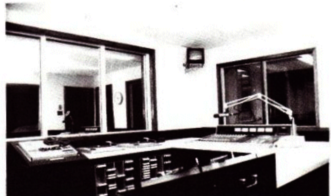
Master Control Room. Another McCurdy 16-channel board handles 2 McCurdy turntables, 2 PR-99 Revox tape machines, local mic, 2 announce booths, 4 Fidelipac playback cart machines through a custom sequencer which will handle up to 8 machines and provides for remote start from satellite control in St. John's to insert local announcements during network operations.
