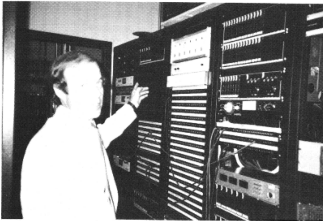
Director of engineering Ted Townsend describes wiring. There are three customized telephone systems: main switchboard is by Mitel; two Bell systems handle contests, using Logic 20 telephones (20 lines), news, using Logic 10s (10 lines).
