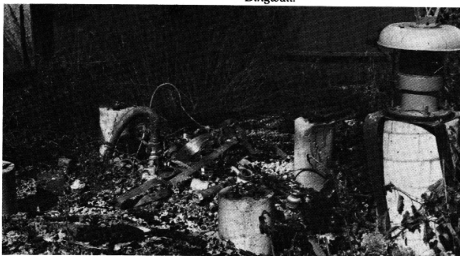
Remains of CFGM Night Array ATU hut, after fire. Photo by Peter May.
