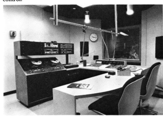
Studio B—also referred to as our 'spoken word' studio—is fitted with a McCurdy custom SS8816 console, two ITC play-only machines, one ITC r/p machine, two Otari reel-to-reel machines, and Technics cassette recorder and turntable. This studio has an adjacent booth fitted with a turret (as in master control). A small turret is fitted on the right of the board, which allows 3-mic interviews. This room is fully self-contained and can be used as an alternate master control.
