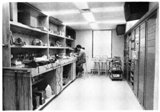
Engineering contains the VHF control and equalization equipment, transmitter remote control and status panel, off-air monitoring, a 30-input/20-output custom switcher by AVL, remotely-operated switchers for selecting control room A or B, delay in/out, processing in/out, satellite receiver, outside temperature, and 24-V DC power supplies for use around the station.
