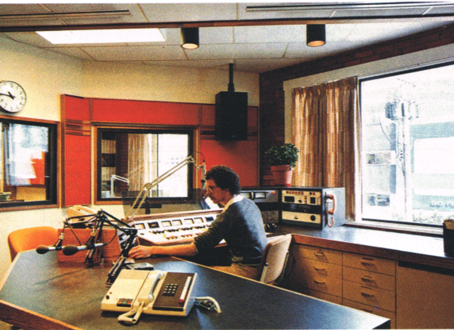
On-air control room. Announcer has view of entrance, news and sports studios. A low-profile design contributes to the spaciousness of the control room. Speakers are mounted from a neoprene isolated "T" hung on ceiling joists. Equipment turret on operator's right contains remote transmitter monitoring, remote status panel, recording input selector panel, remote control room switcher, temperature indicator, intercom, PA and front door control, and a cassette deck.
