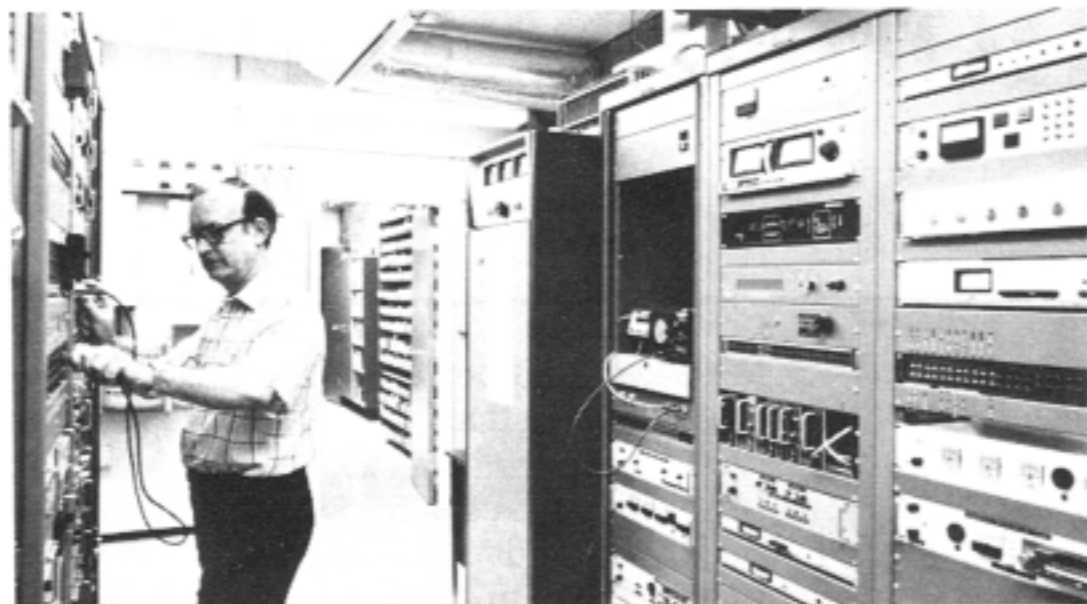
Assistant engineer Dave Shearer in C-FAX rack equipment area. Rack in foreground is alternate STL equipment; next contains all transmitter status equipment; third, adjacent to RCA emergency transmitter, contains transmitter control equipment.
