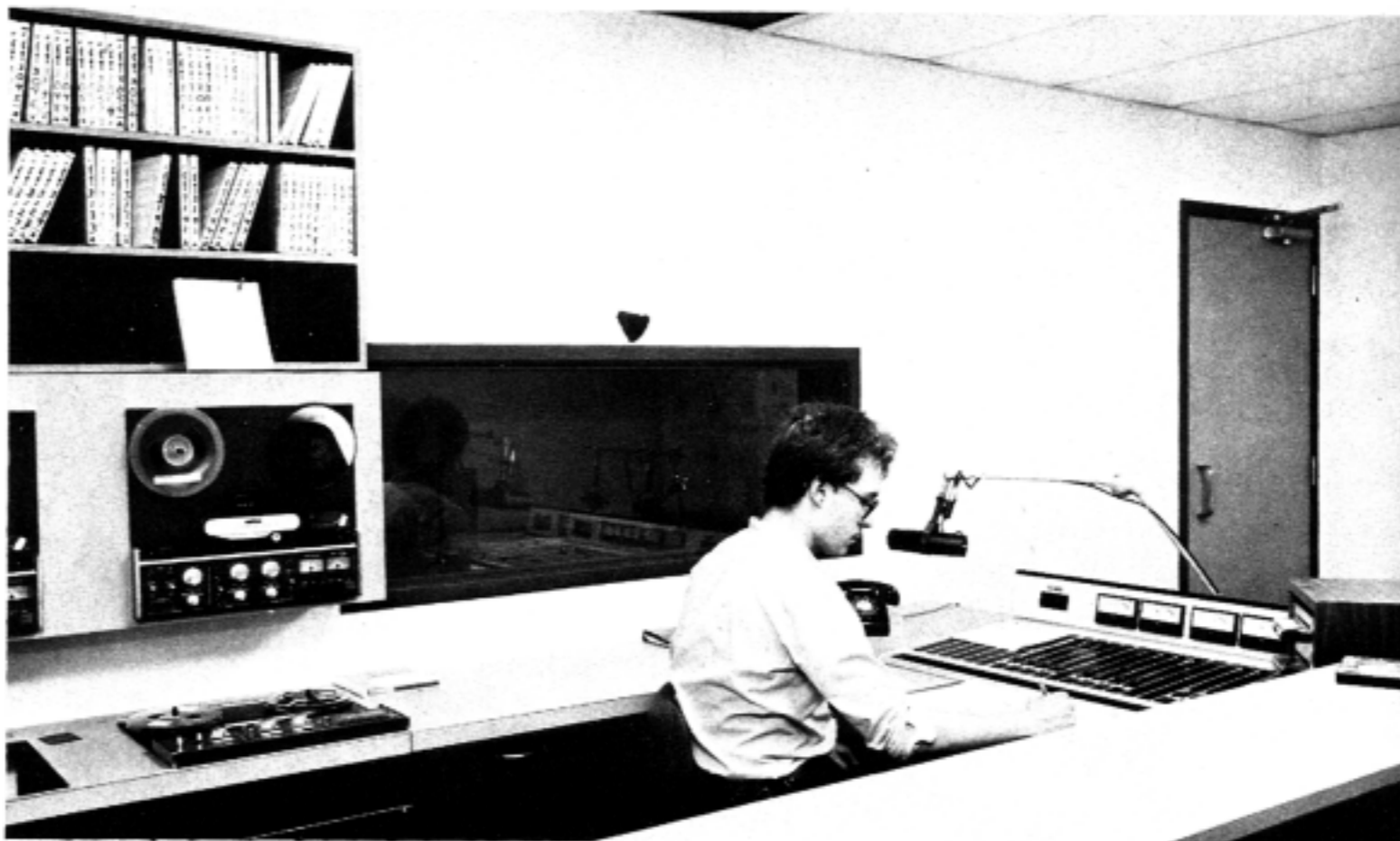
CJMX-FM master control is equipped with Ward-Beck board, three Studer Revox B77 stereo tape machines, two Technics turntables, an Ampro three-cart machine and Shure microphone. Station uses CCA 20 kw transmitter, complete with Optimod, and 12-bay antenna is mounted on Mid-Canada Communications tower, shared by CICI-TV and CIGM-FM.
