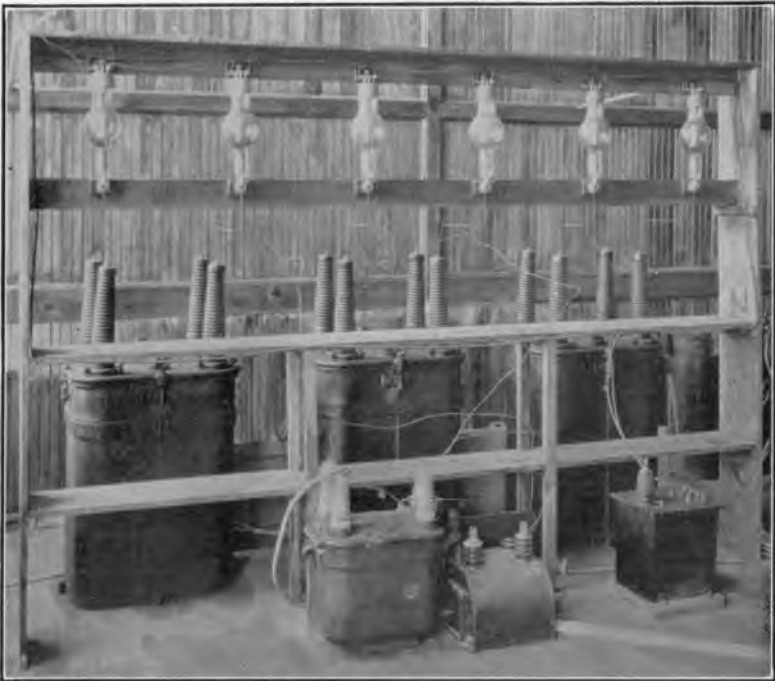
FIGURE 151.—Kenotron rectifier set, 20 kilowatts.
