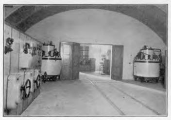
FIG. 192.-Jannowitzbruecke substation of Berlin elevated railway.
