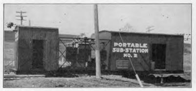
FIG. 200.-Exterior view of Calgary portable rectifier substation.
