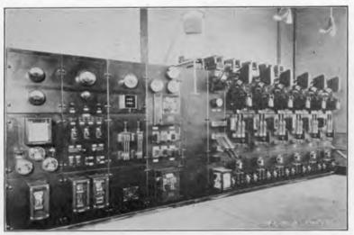
FIG. 181.-Control switchboard in Maypole substation.
