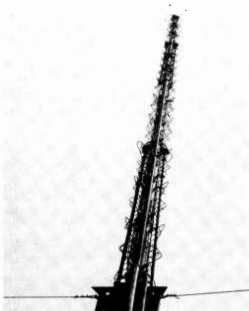
Fig. 13-9. Typical bat-wing antenna.
