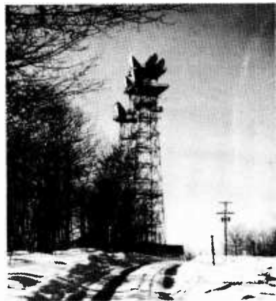
Fig. 1-27. Microwave relay station at Green Pond, N.J.
