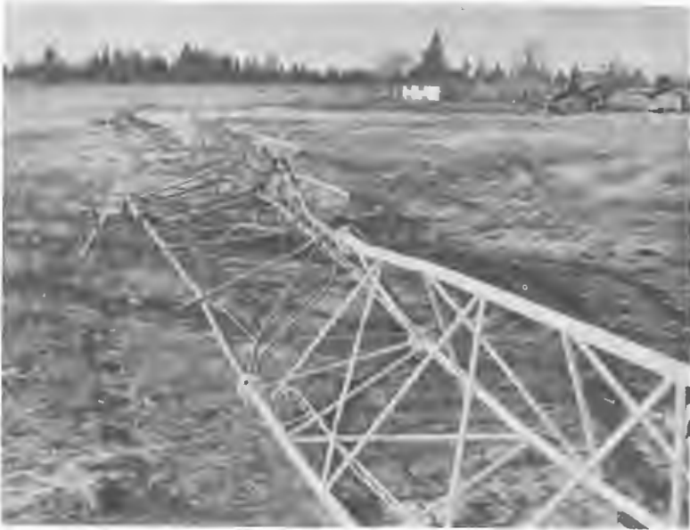
Figure 30.12 Wreckage of mast top sections (Courtesy KHQ)
