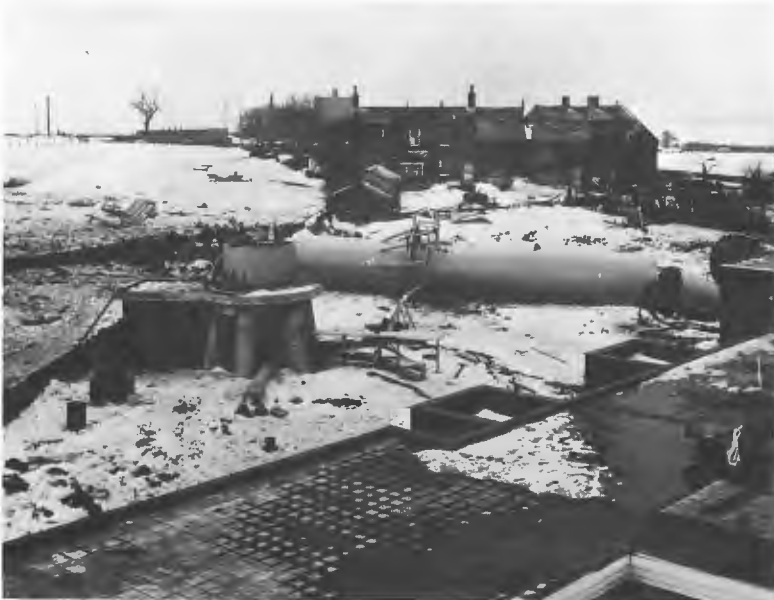
Figure 43.19 Base segment and superstructure after collapse of structure (Courtesy Construction News)
