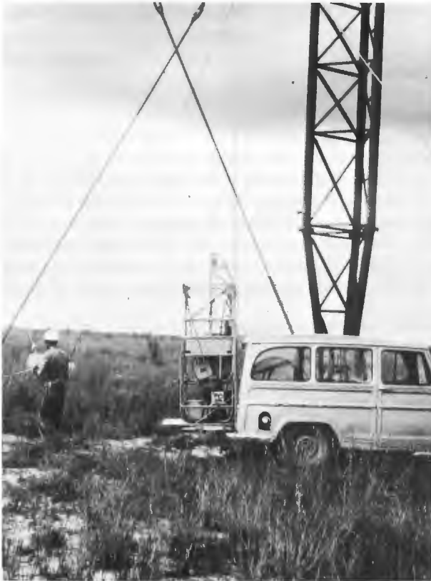
Figure 26.1 Mechanically driven work box for curtain antenna maintenance
