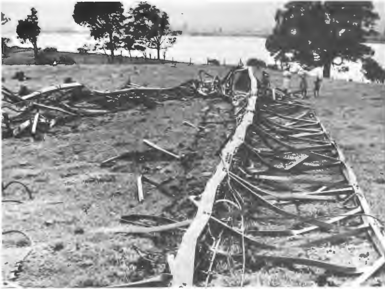
Figure 43.6 U shaped distribution of mast wreckage
