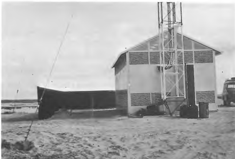
Figure 43.24 Protective fence to prevent erosion
