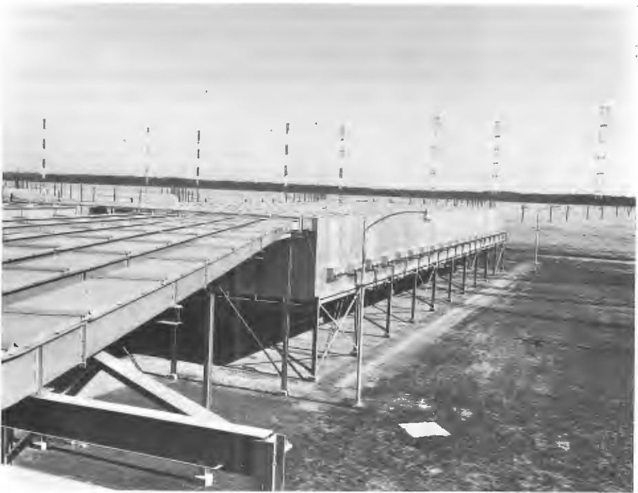
Figure 27.2 Shielded transmission line and switching matrix (Courtesy Continental Electronics)
