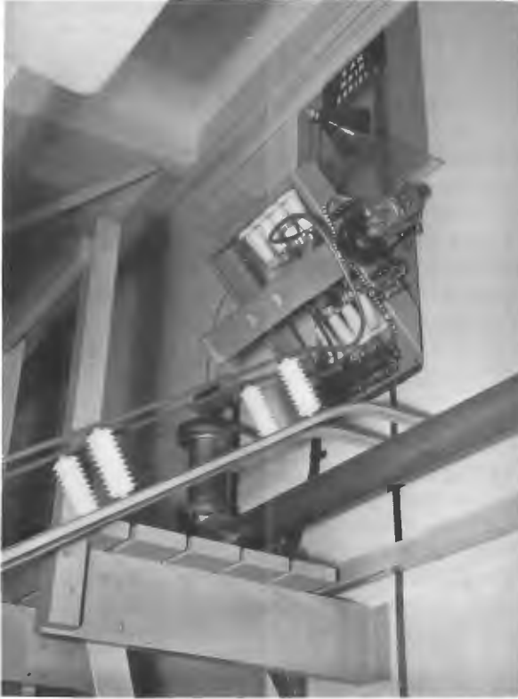
Figure 41.5 Rotary switch with rubber tired wheel
