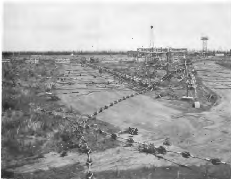
Figure 20.2 Damage to antenna system resulting from cyclone
