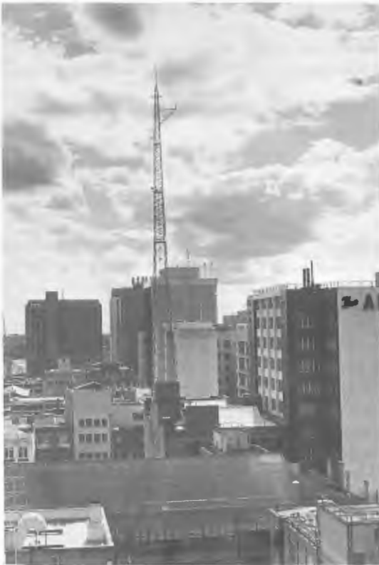
Figure 44.1 Base insulated broadcast antenna on city building
