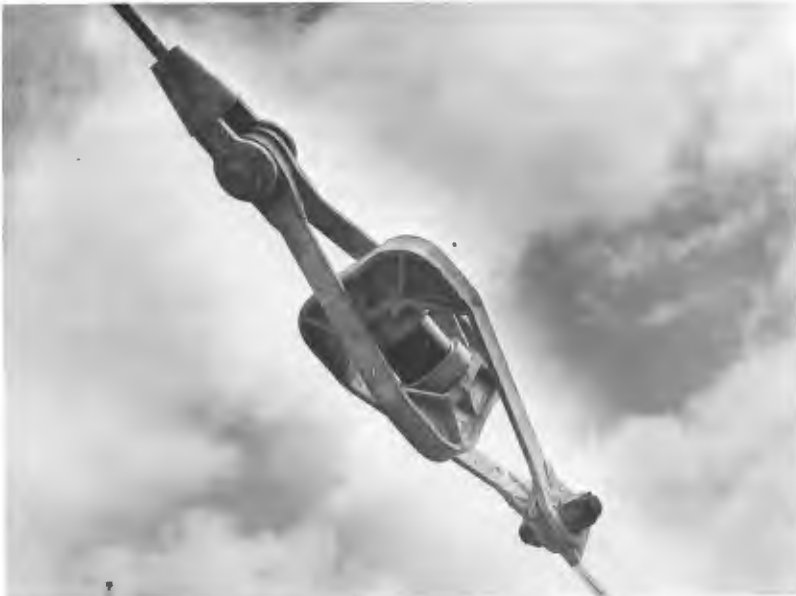
Figure 38.5 Solid type guy insulator
