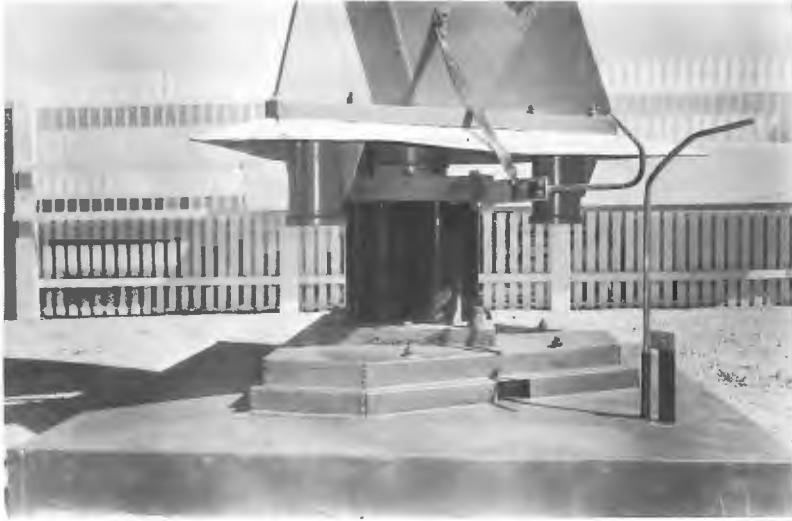
Figure 38.8 Typical horn gap installation
