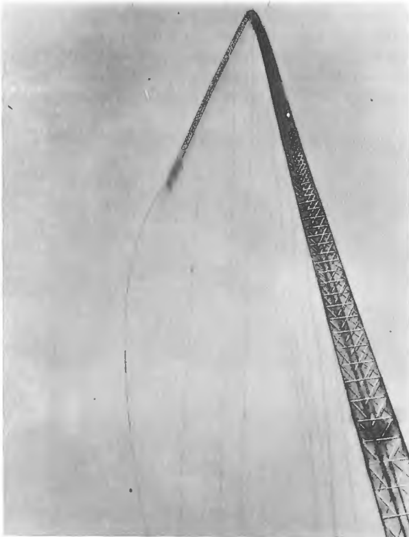
Figure 30.8 Top section falling (Courtesy WMT)
