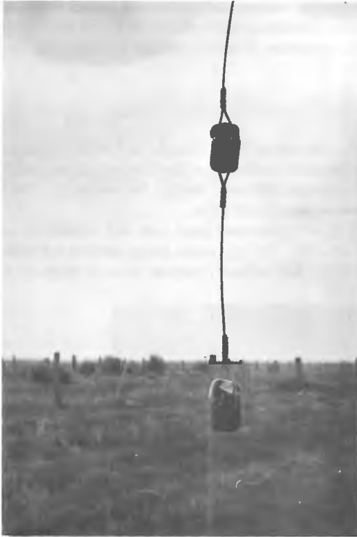
Figure 43.18 Damaged dipole termination
