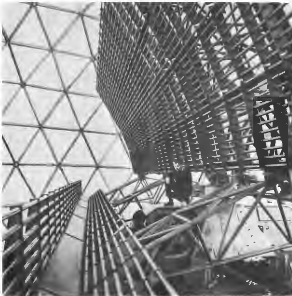
Figure 25.2 Typical airport radar installation (Courtesy The Marconi Co.)
