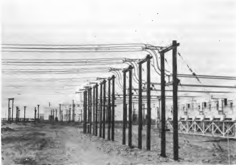
Figure 41.9 Pressure treated transmission line poles
