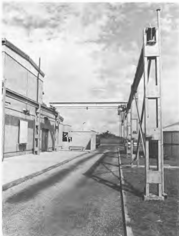
Figure 30.1 Gantry for material handling
