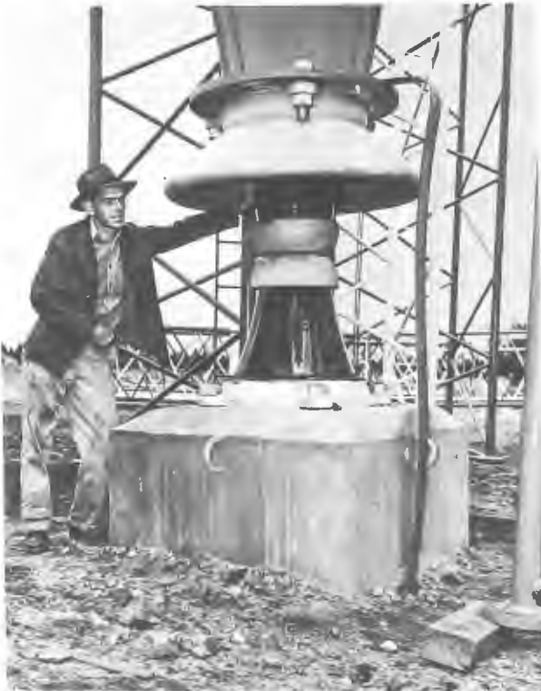
Figure 49.1 Erection of mast radiator (Courtesy KHQ)
