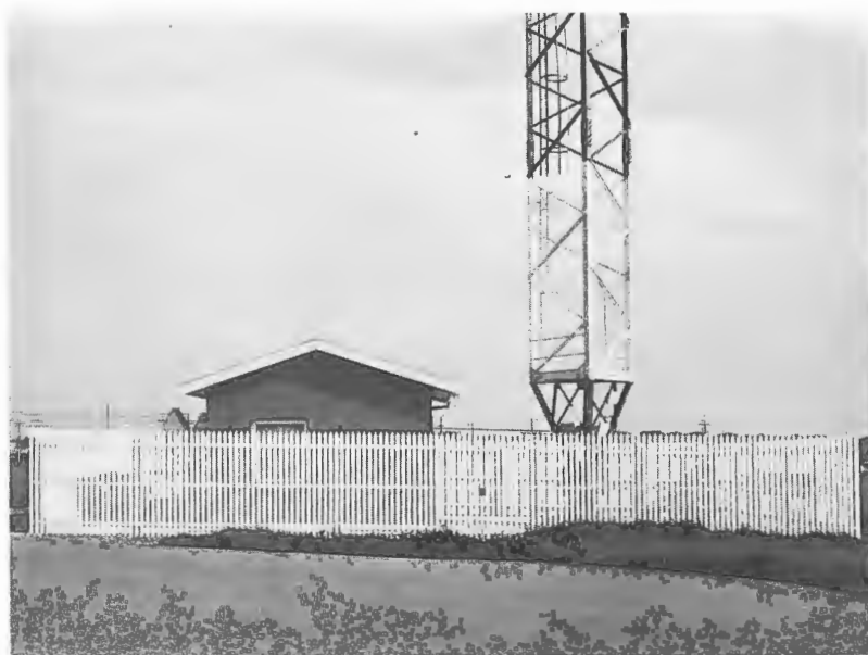
Figure 27.6 All wood type security enclosure
