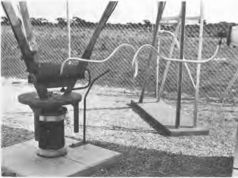
Figure 38.9 Series inductor
