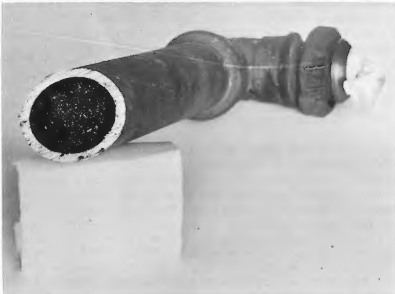
Figure 42.2 Sediment in copper piping of water cooling system
