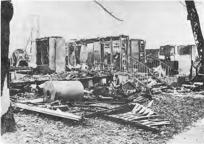
Figure 34.2 Building and equipment damage (Courtesy Leo Forster)
