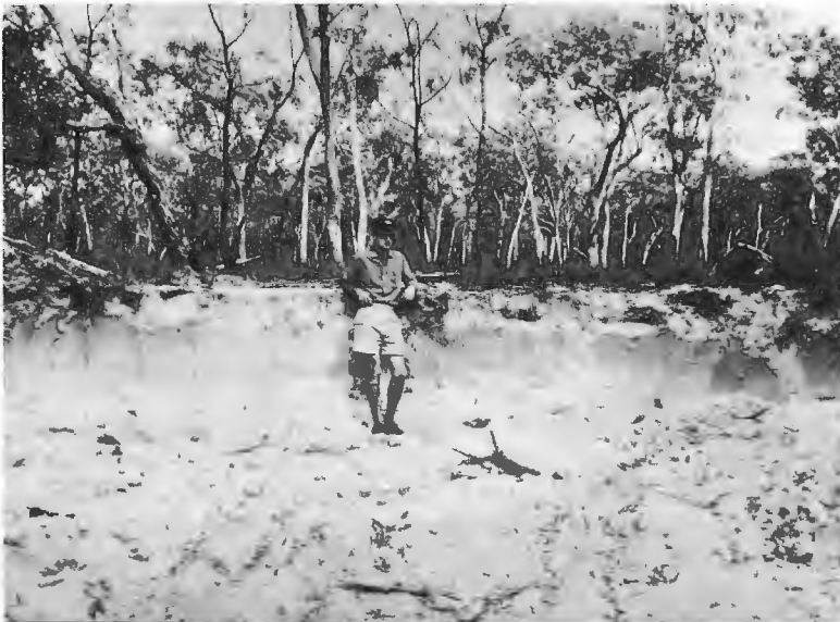
Figure 41.11 Sand pit for remote station construction
