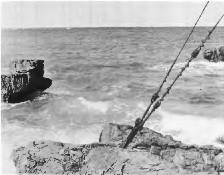
Figure 26.9 Guy anchor near the sea (Courtesy Far East Broadcasting Co.)
