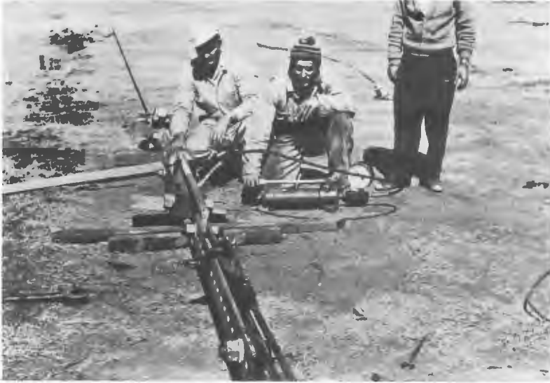
Figure 48.6 Pretensioning a guy rope prior to erection
