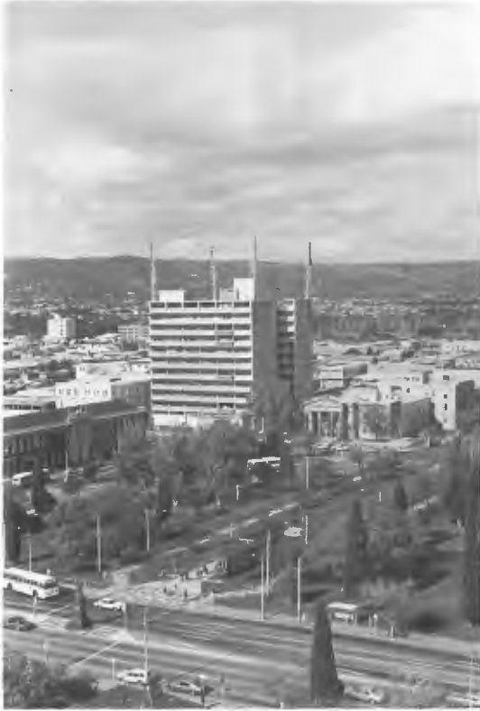
Figure 44.5 Roof top antenna and support structures
