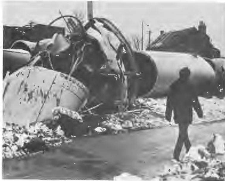
Figure 43.22 Buildings damaged by falling steel and guy ropes (Courtesy Construction News)
