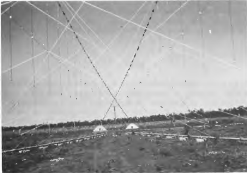
Figure 41.7 Plastic ropes used to maintain antenna stability
