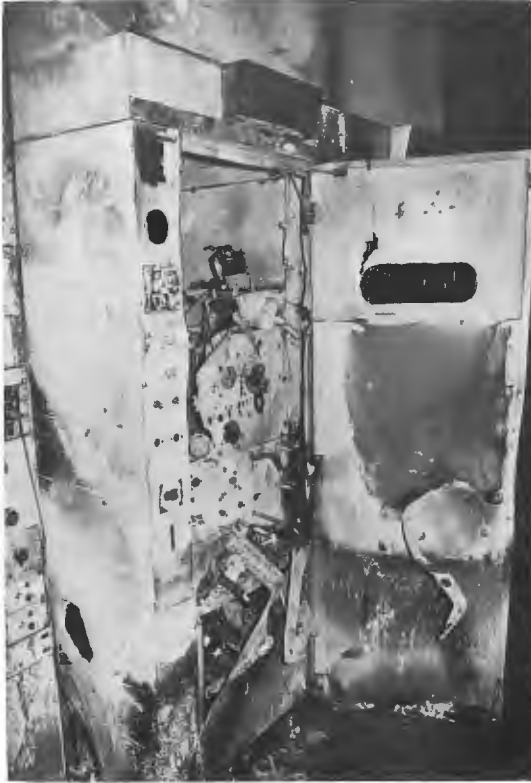
Figure 33.1 Sheet metalwork damaged by fire
