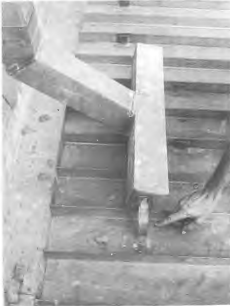
Figure 47.3 Roof bonding at 250 kW station
