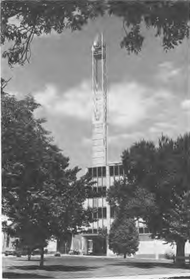
Figure 44.6 Microwave antennas and structure on city building
