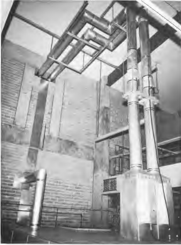
Figure 27.3 Bonding and earthing strap for transmission line
