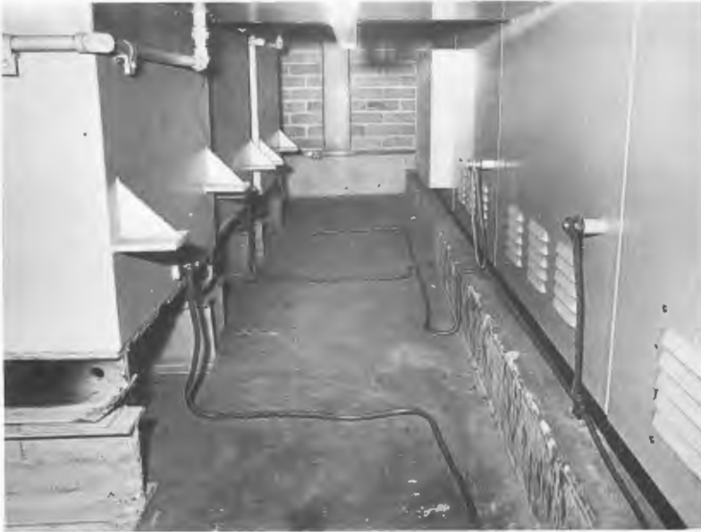
Figure 28.2 Stepped vault floor to contain oil spread
