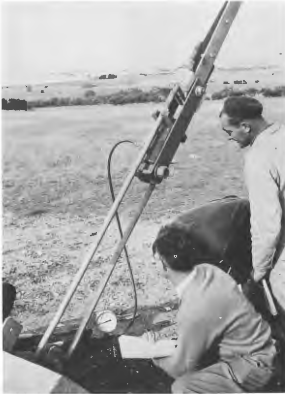
Figure 43.25 Equipment used to measure guy tension
