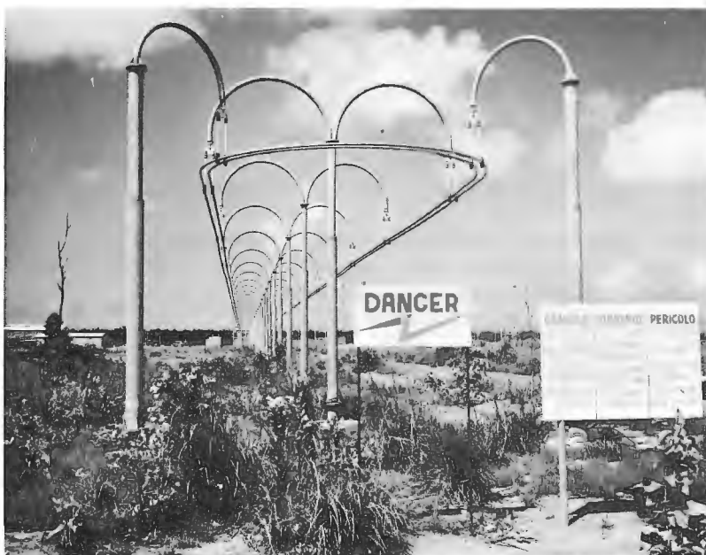
Figure 22.1 Danger notice near dissipative line
