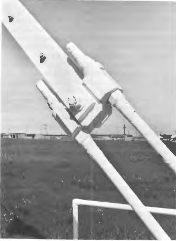
Figure 41.10 Guy anchor rod thread protection
