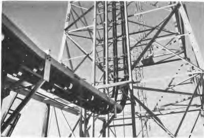
Figure 38.1 Clamping and bonding of insulated waveguide
