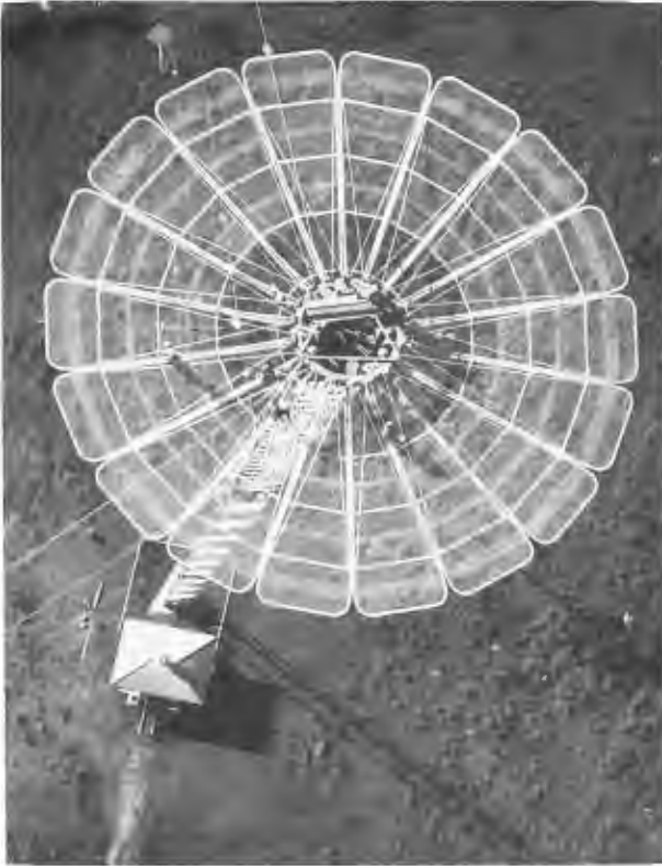
Figure 15.4 Dual frequency radiator 198 m high fitted with 18 m diameter armature (Courtesy Courier Mail)
