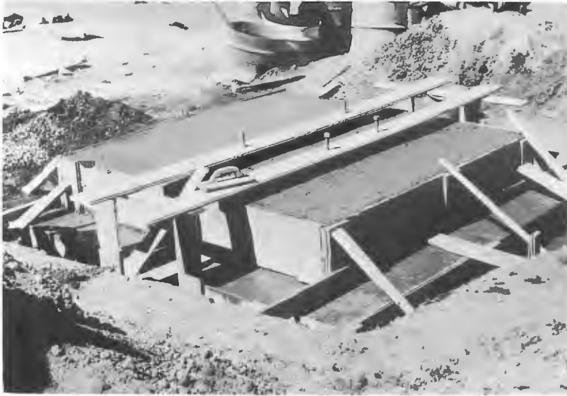
Figure 48.5 Mast thrust block prior to trowelling-off
