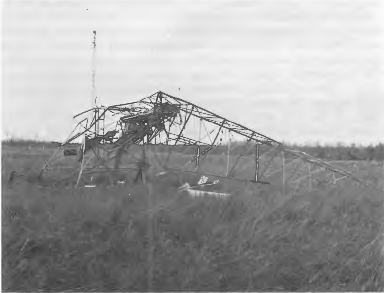
Figure 43.16 Collapsed standby antenna
