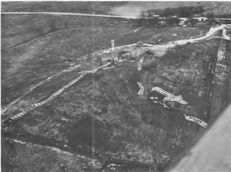
Figure 30.9 Mast wreckage on the site (Courtesy WMT)
