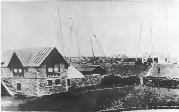
Figure 43.5 Damage to antenna (Courtesy Marconi Wireless Telegraph Company)
