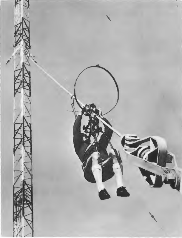
Figure 26.4 Bosun's chair guy inspection device
