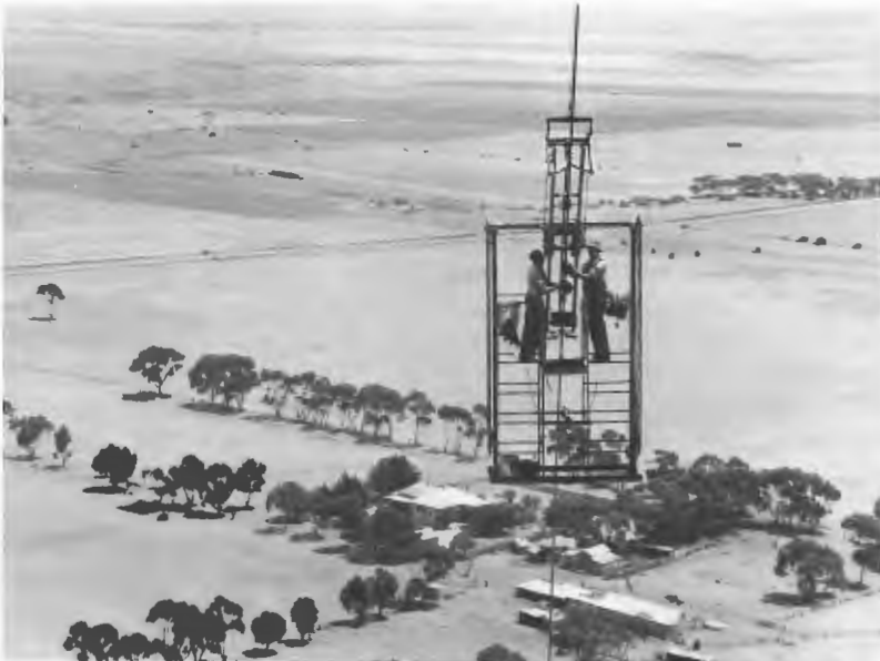
Figure 26.3 Guy inspection cage
