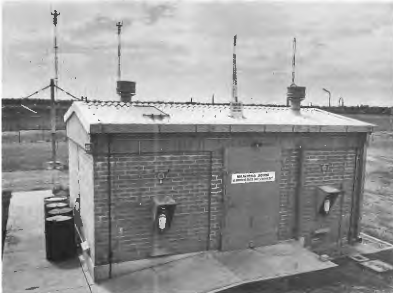
Figure 33.3 Flammable liquid store
