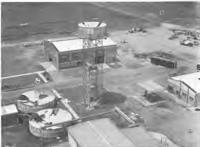
Figure 40.4 Damage to buildings and water supply facilities
