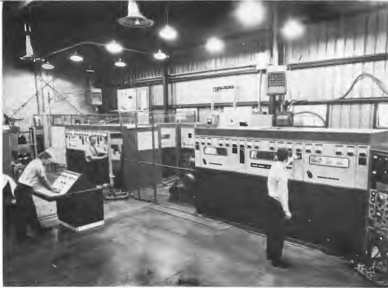
Figure 48.2 Factory tests being conducted on 200 kW m.f. transmitters (Courtesy Continental Electronics)
