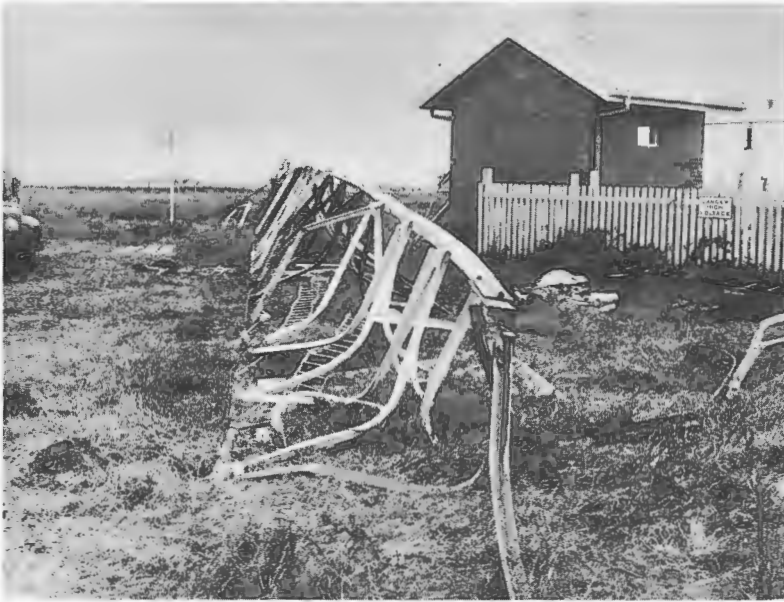
Figure 26.15 Damaged section near main antenna matching equipment building
