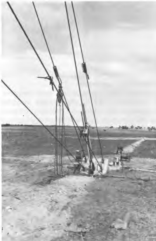
Figure 30.2 Typical anchorages required for safe mast erection
