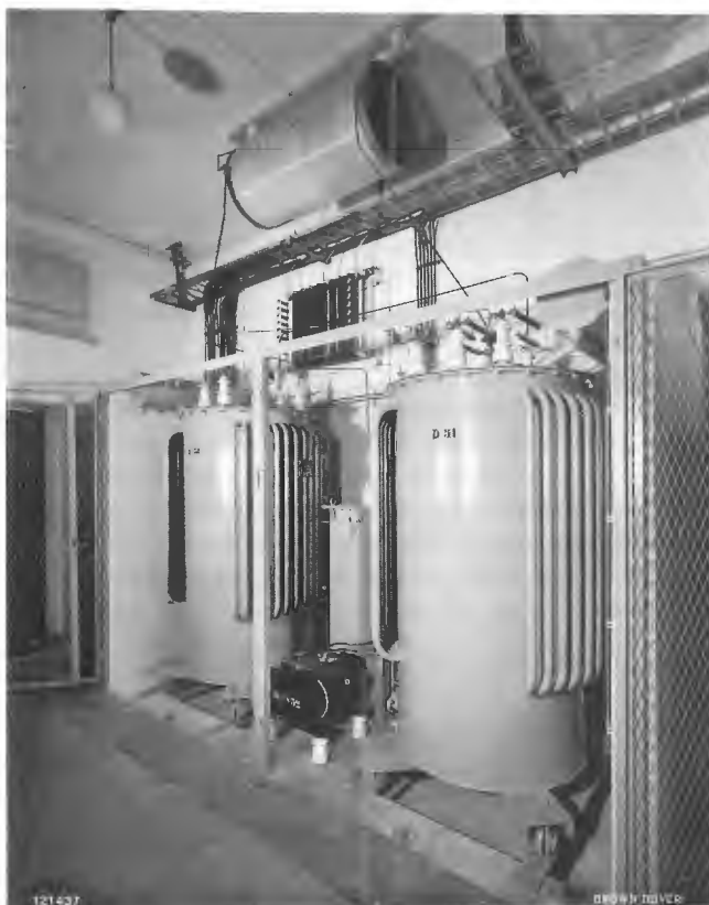
Figure 36.2 Modulation transformer and reactor of 250 kW m.f. transmitter (Courtesy Brown, Boveri and Co)
