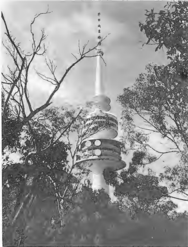
Figure 44.9 Telecommunication tower, Black Mountain (Courtesy The Canberra Times)
