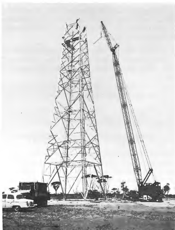
Figure 30.4 Use of crane for tower erection
