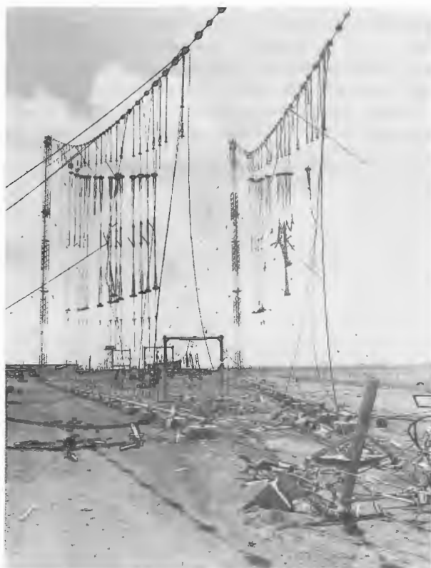
Figure 43.14 Damaged antenna elements
