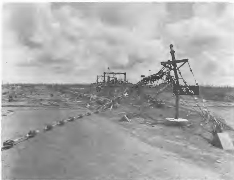
Figure 43.13 Collapsed log-periodic antenna
