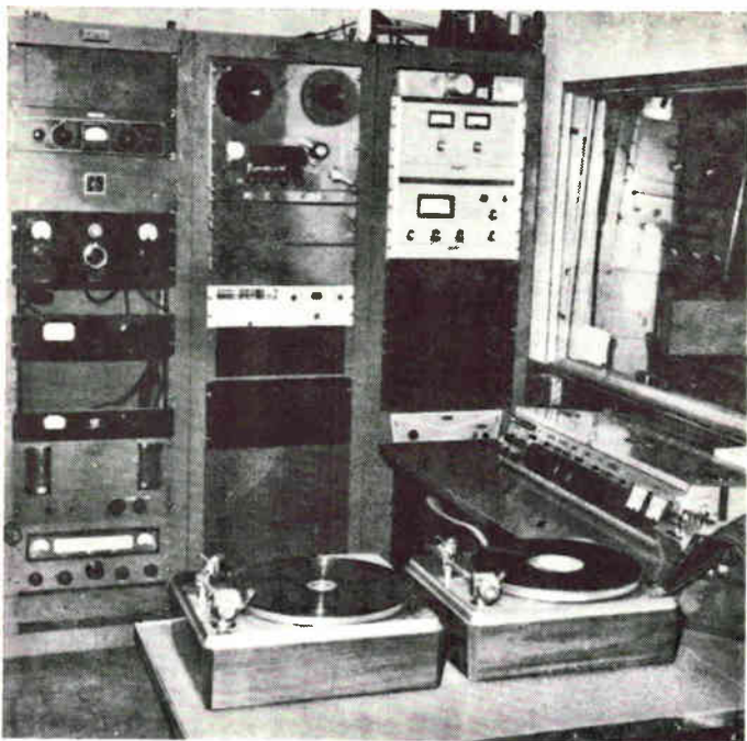
Transmitter-site studio. The racks contain both AM and FM monitoring equipment and other necessary terminal gear. The operator faces the transmitters through the large double-paned window.
