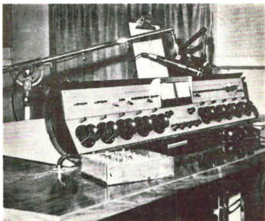
Fig. 2. Two views of the WAJR-FM production area. Rack equipment is in close proximity.
