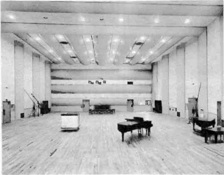
Fig. 2-66B. Rear view of Republic Corporation scoring stage showing polycylindrical diffusers on rear wall and ceiling.
