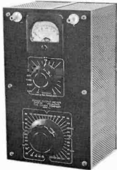
Fig. 10-35A. A power-output meter manufactured by the Daven Company.
