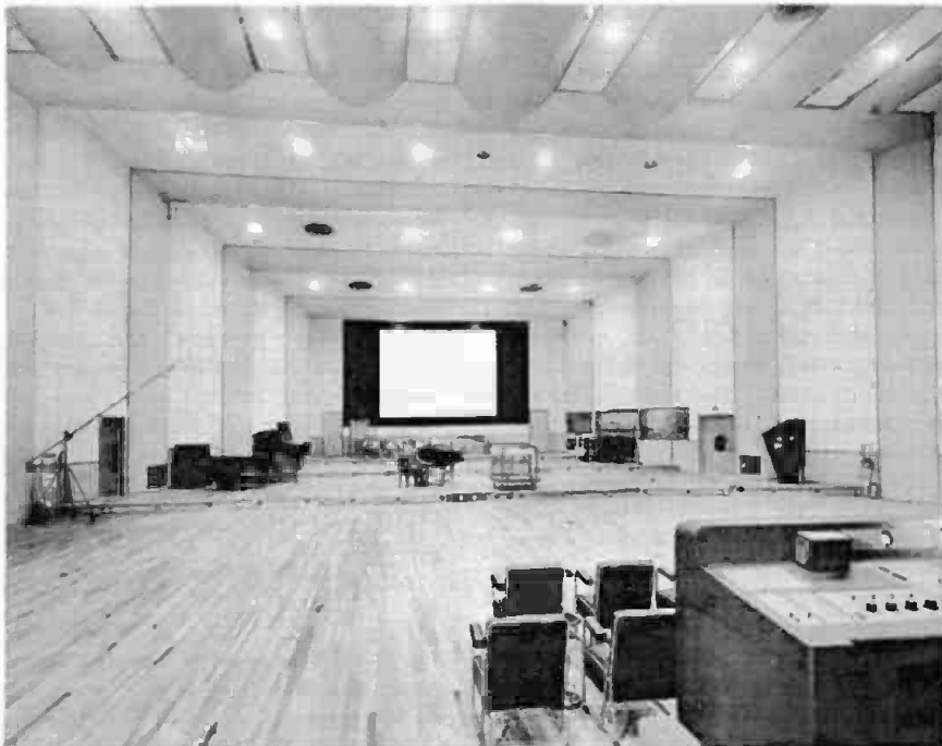
Fig. 2-66A. View of Republic Corporation scoring stage looking toward the screen. Polycylindrical diffusers may be seen along the sidewalls and on the ceiling.
