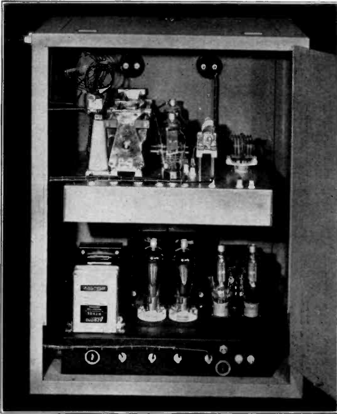
Figure 14. REAR VIEW OF R.F. AMPLIFIER AND MODULATOR.
