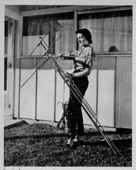
Fig. 46-First step in the installation is assembly of the antenna mast and lead-in wire to the ground, as shown in this photo by the Winegard Company. This Winegard antenna is a "jiffy-rig" type which unfolds like an umbrella.
