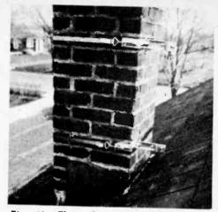
Fig. 49—The chimney mount wraps around chimney, requires no screws to be put in or holes to be drilled.
