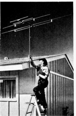
antenna in bringing in to the set a strong, clear signal. Without such a signal, the set cannot operate properly. Snow, ghosts, interference, dim pictures and unstable sync (vertical rolling and/or horizontal tearing) are but a few of the troubles which may result if a strong, clear signal is not present at the set's antenna terminals. 5
