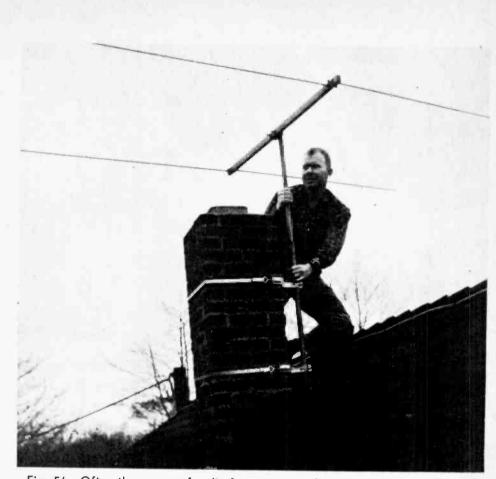
Fig. 56—Often the source of radio frequency interference can be "tuned out" by orientation of the antenna.
