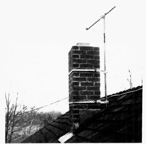
roof 15 to 20 feet high, any mast up to 8 feet long would be sufficient out to about 25 miles. From 25 to 50 miles, 12 feet (above the house) might be enough. Beyond 50 miles 20 feet and more is customary. At great distances, it is not uncommon to put up a small "tower" on the house or next to it, with heights (overall) of 100 feet.
