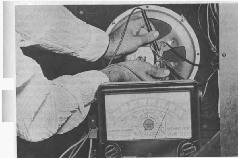
Fig. 11-4. Testing continuity of speaker field.
