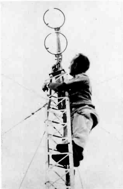
Fig. 2-15. Antenna Installation at United States Air Force TV Station, CSL-TV, Azores. The Rings are Separately Excited from Aural and Visual Transmitters. Official United States Air Force Photo.
