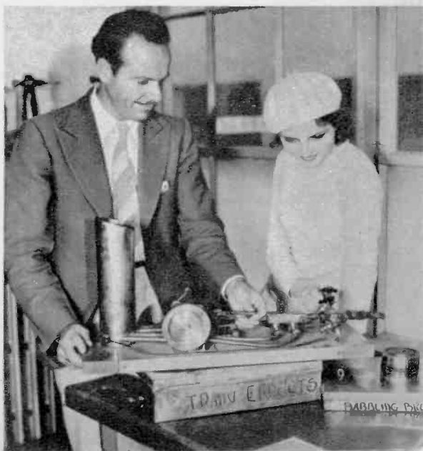
This contraption of cogs and valves was used for train noises in one of the first sound movies at Warner Bros. studios. Sound on film is at right.
