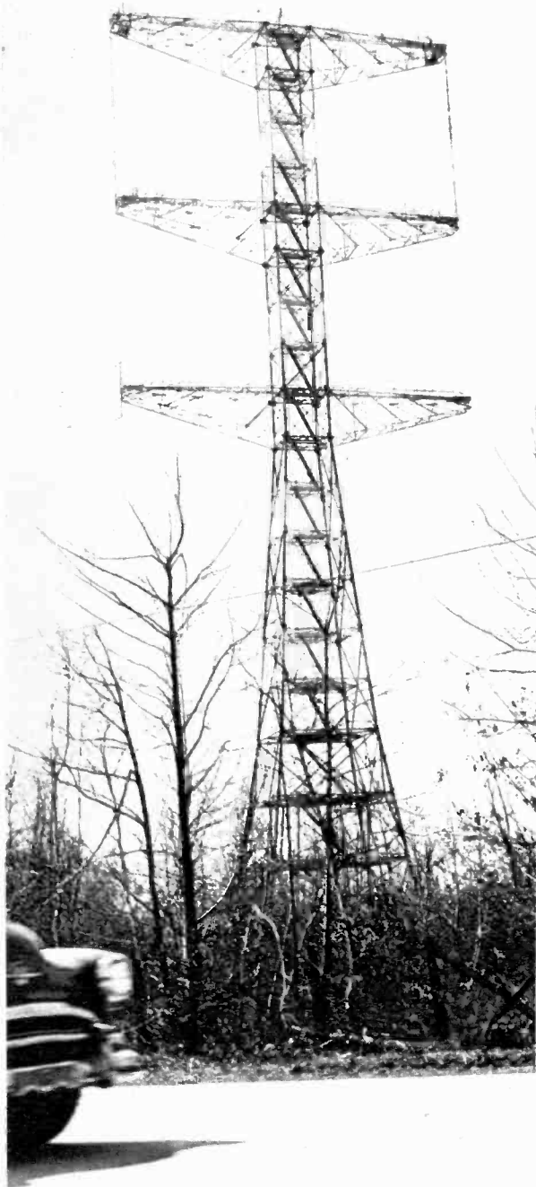
Major Armstrong's experimental transmitting tower on the Hudson palisades near Alpine, New Jersey, is 400 feet high and 1,000 feet above sea level.
