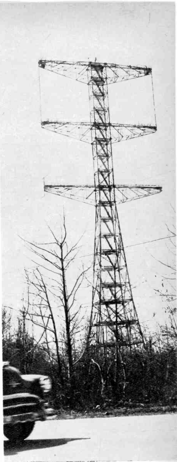
IN 1937, Armstrong built this experimental transmitting tower on the Hudson palisades. It is 400 feet high and 1,000 feet above sea level.
