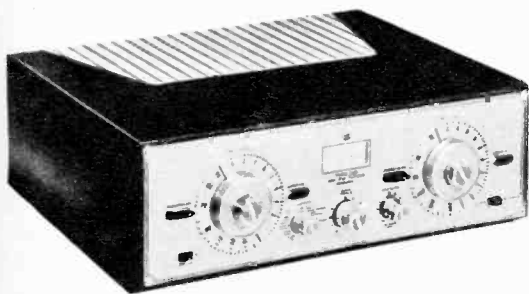
STEREO can be economically added to existing high-fidelity systems with the Bogen ST10. Dual preamp, 10-watt amplifier are in the one unit.
