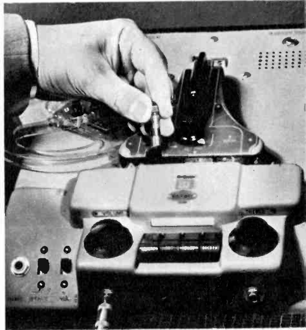
SOME CAPSTANS have threaded mounts, permitting easy removal for changing speed, cleaning.
