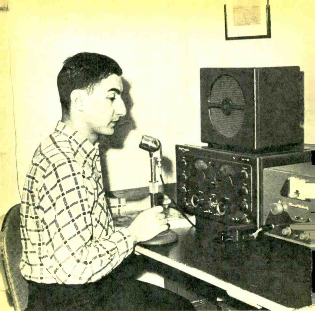
Station K2DUX. Equipment includes the DX-40 with mike and key, and a NC-183D receiver.
