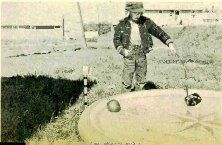
Installation of alarm. Adjust float arm so that slight water rise will not ring bell.
