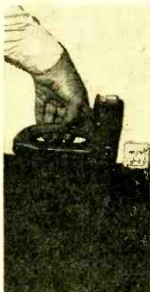
Telephone extension jack is mounted on baseboard near desired location of remote unit.
