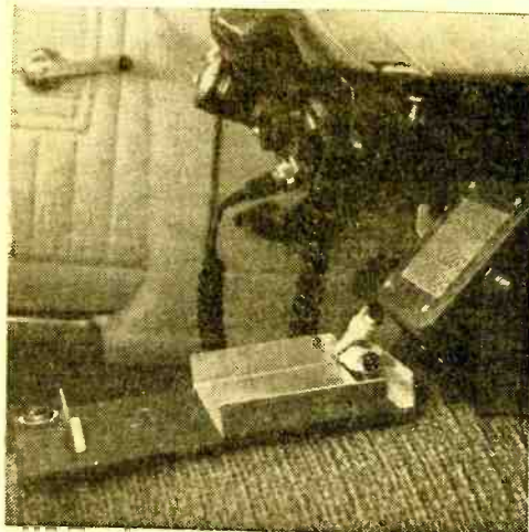
Bracket on transmission hump is ready for installation of recorder. Connector cables underneath are fastened to Masonite with a cable clamp. This prevents any strain on connector's terminals. Speaker at right and mike above are for two-meter mobile rig.
