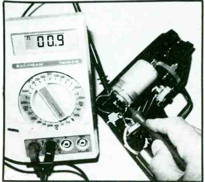
Figure 14: Check the motor continuity when normal battery voltage is measured at the motor terminals.
