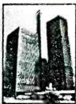
Germany Radio Broadcast Center Federal Republic of Germany
