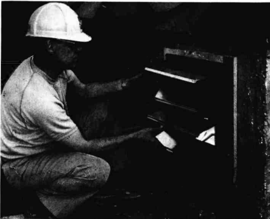
Check the operation of the self-opening louvres. Be sure that they do not bind, scrape or stick. Remove any bits of material that might cause sticking, after all you want to make certain they open everytime. Who wants to go on the roof more than they have to?
