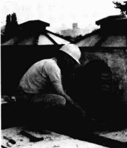
Don't let stray nails or fragments lie about on the roof. If you step on one, then there goes your roofing materials!
