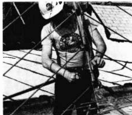
Secure the antenna to the mast. Most damage to the elements occurs at this time.
