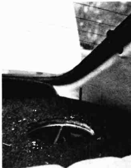
Fig. 6. Cut a hole in the rear deck cover corresponding to the cutout in the steel deck underneath.
