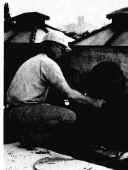
A stud and interior plaster had to be removed. We hammered away splinters and used an old drill bit to do the remainder.
