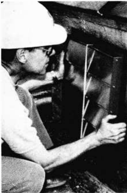
The fan fits! However, thermostats must be secured to the inside of the air duct and a wood frame made to support the fan.
