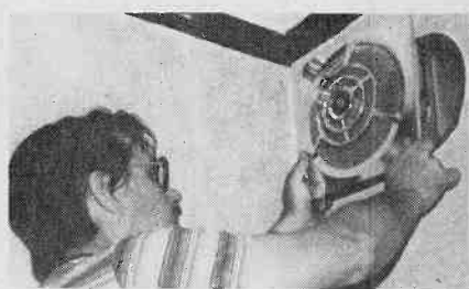
Fig. 15. After the fan is checked out for operation and multi-speed control (if so equipped), install the automatic damper doors and grille on the inside. Be very careful not to bend or force the damper doors into the duct. Make certain the dampers swing open at all settings of the fan's multi-speed control. The wire screen should be removed periodically for cleaning. Don't wait too long; if you do, you'll be wasting valuable electricity.
